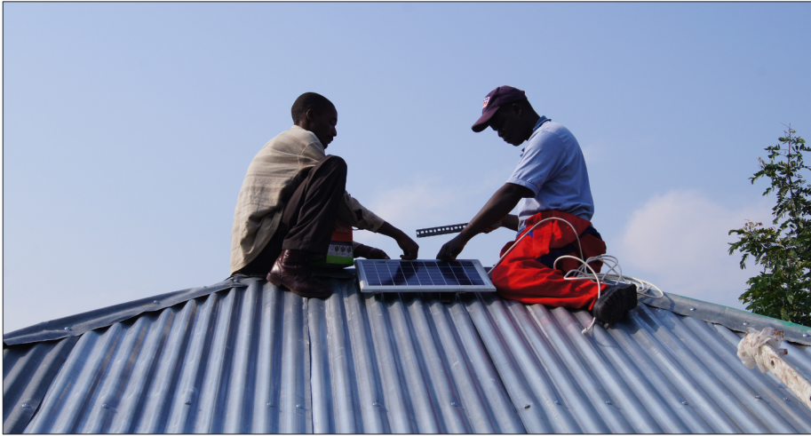
Solar panel installation, Rusinga Island, Kenya; Alexandra Hiscox
