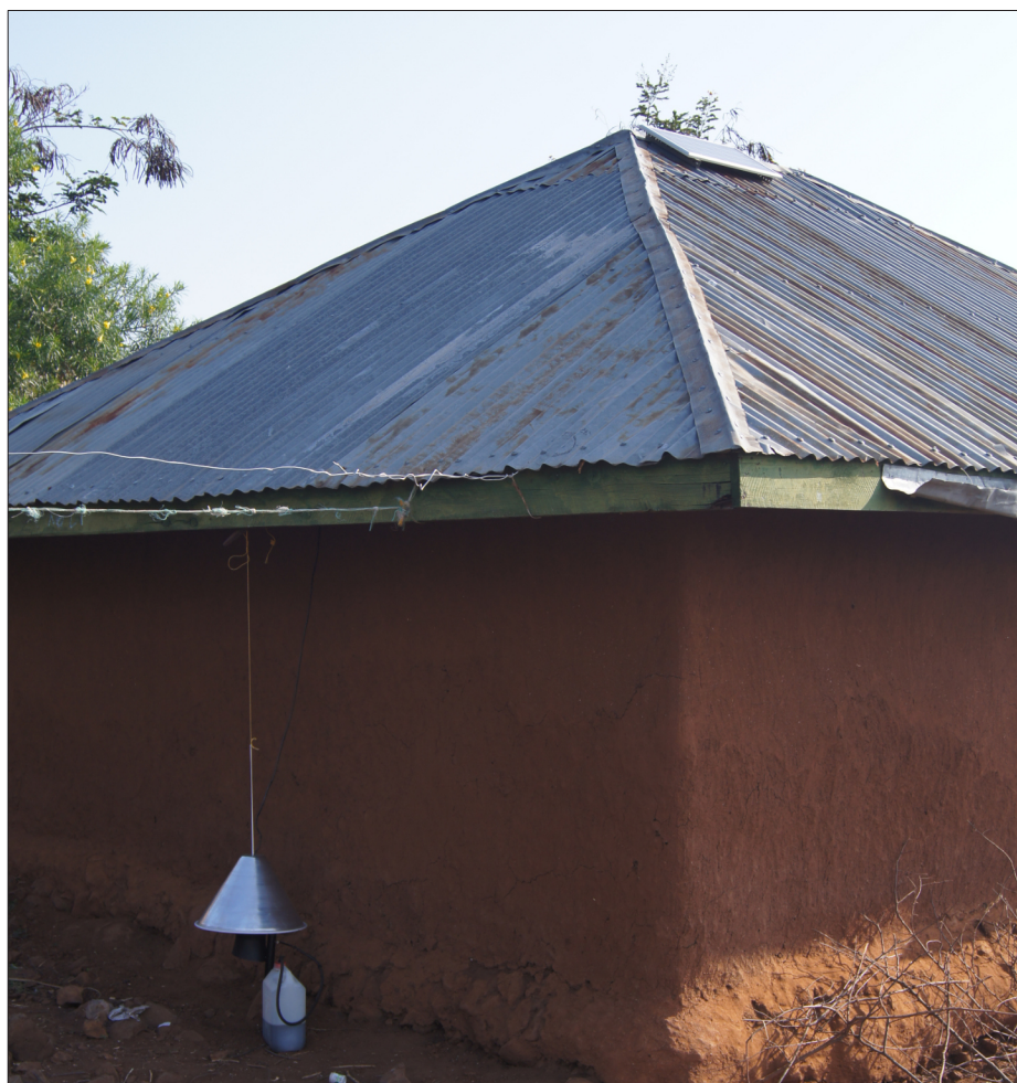
Solar panel on roof of house in Kenya; Alexandra Hiscox
